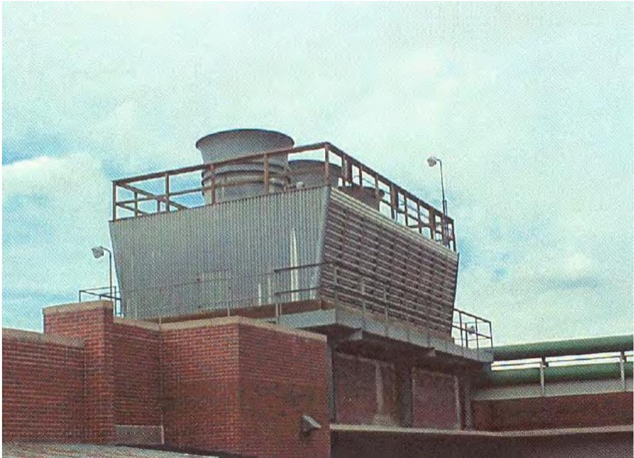
Figure 7 Cross-flow cooling tower
